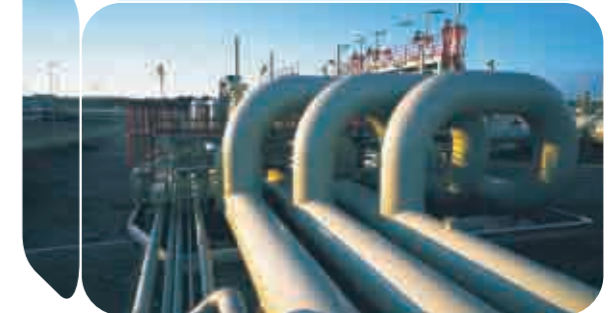
West- east gas pipeline
