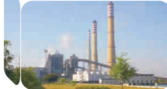
Thermal power plants
